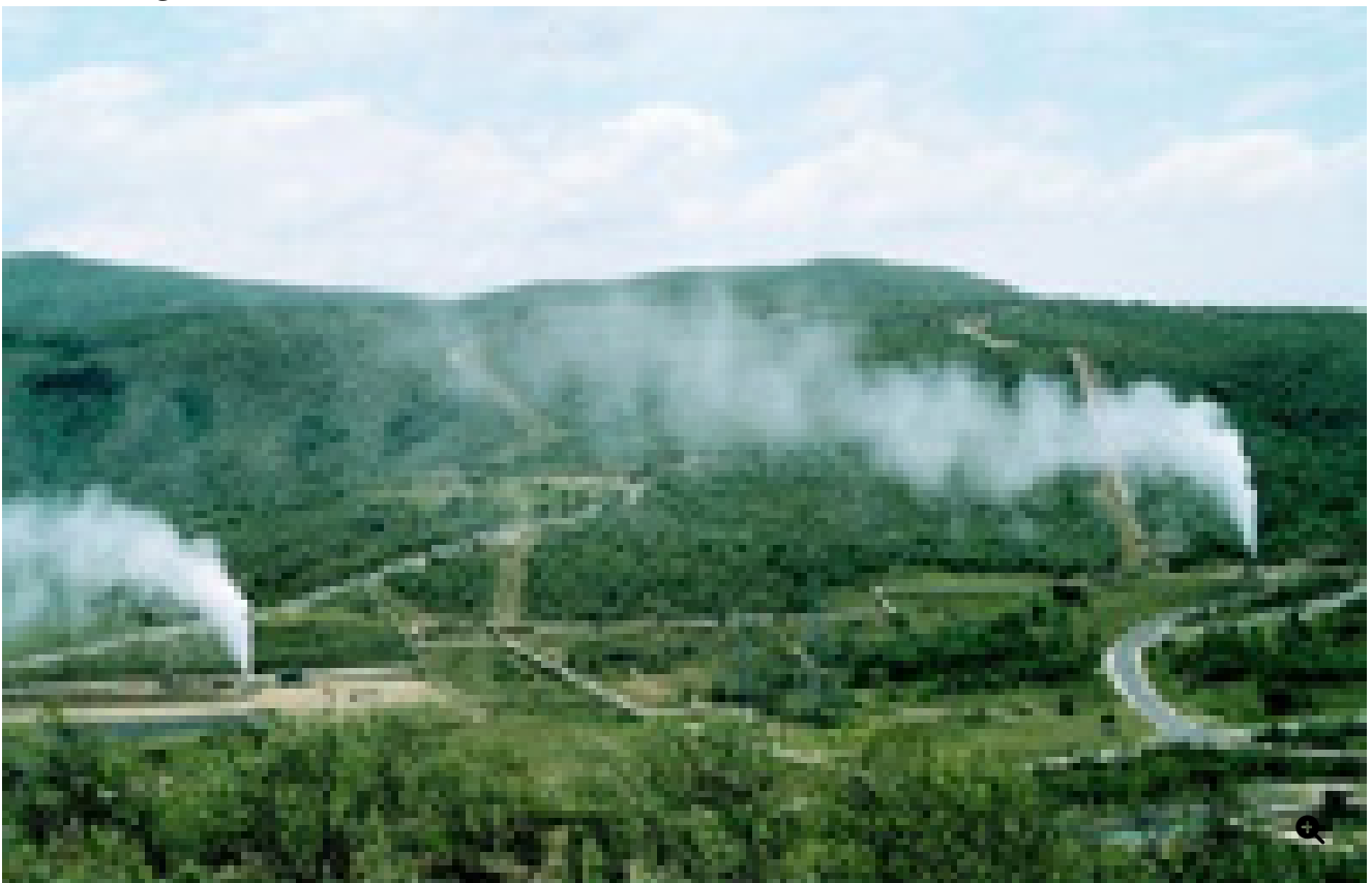
The Olkaria plant in Kenya's Rift Valley
